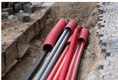
Regular Waste Pipe
